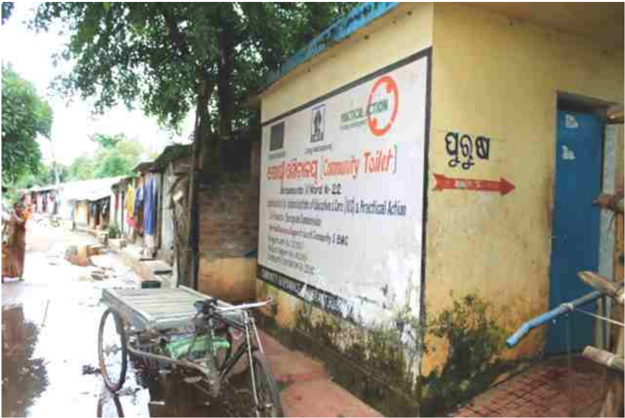
Community Toilet in Birsa Munda Slum, Bhubaneswar
